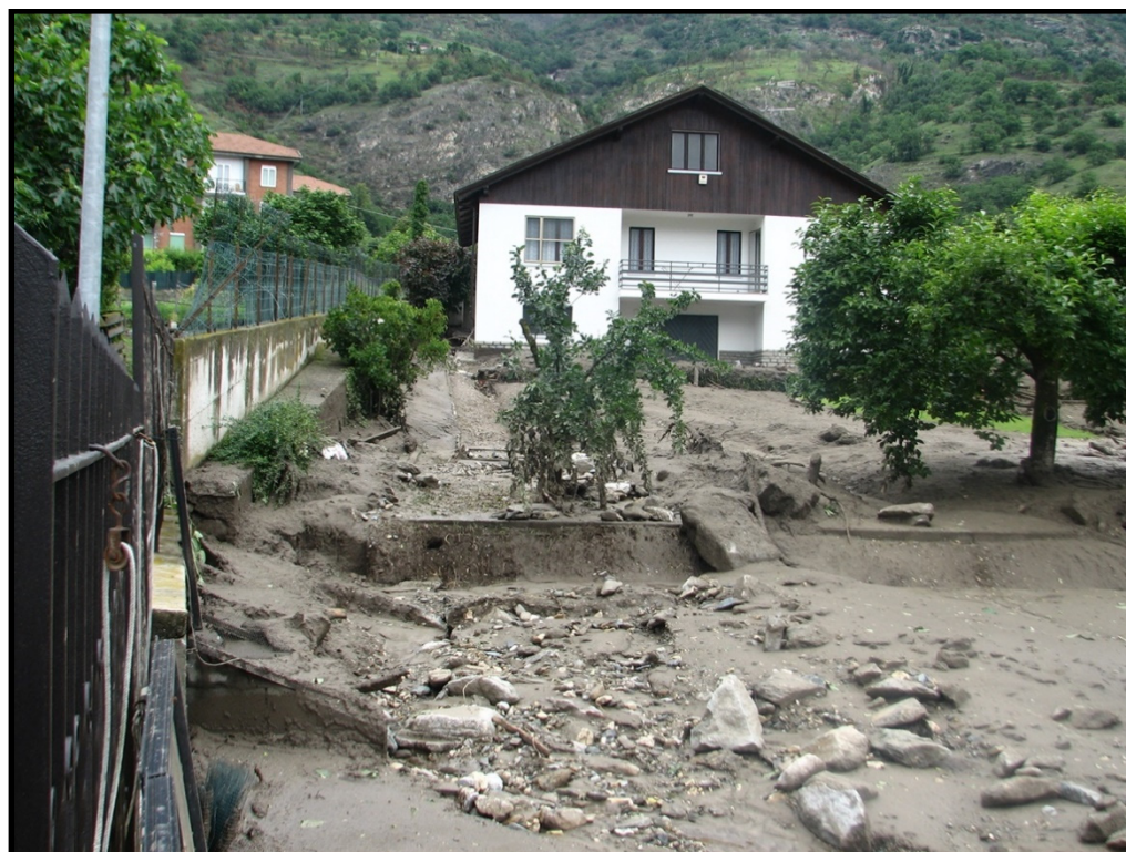
Figure 5. Debris flow deposits involving buildings in Bussoleno municipality.
