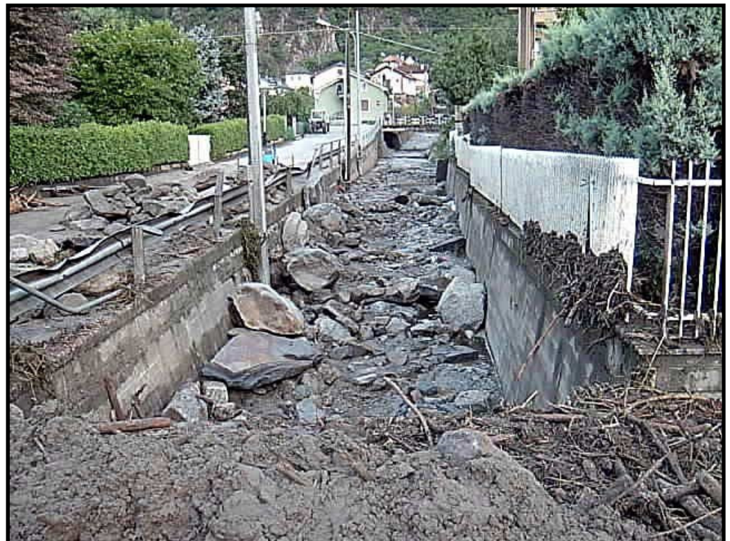
Figure 2. Debris flow deposit in channel bed.
