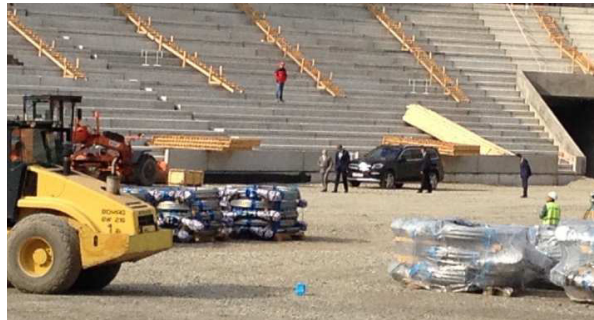
Fig. 10. Site Preparation with Reinforced wooden strips.
