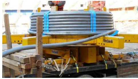
Fig. 9. Redaelli Cable on the uncoiler.
