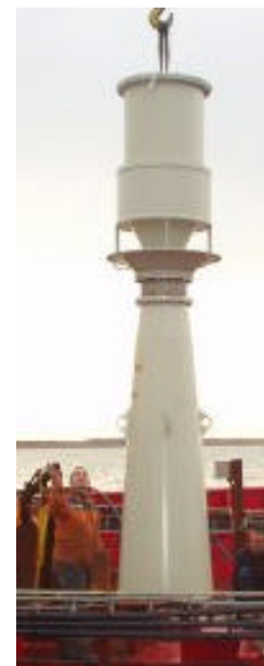
Figure 9: The six axial propeller turbines being assembled at Kössler GmbH (left) and one of the turbines being installed on the prototype in open sea
