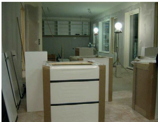
Figure 1: Kitchen installation in a volume element
