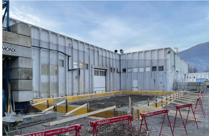
Figure 2. Concrete diaphragms, 13.5 m deep, define the rectangular well
