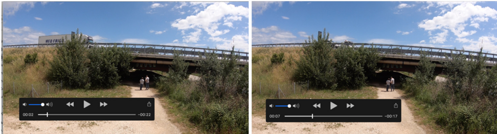
Figure 9: Vibrational test of a steel seismic restrainer of the bridge.
