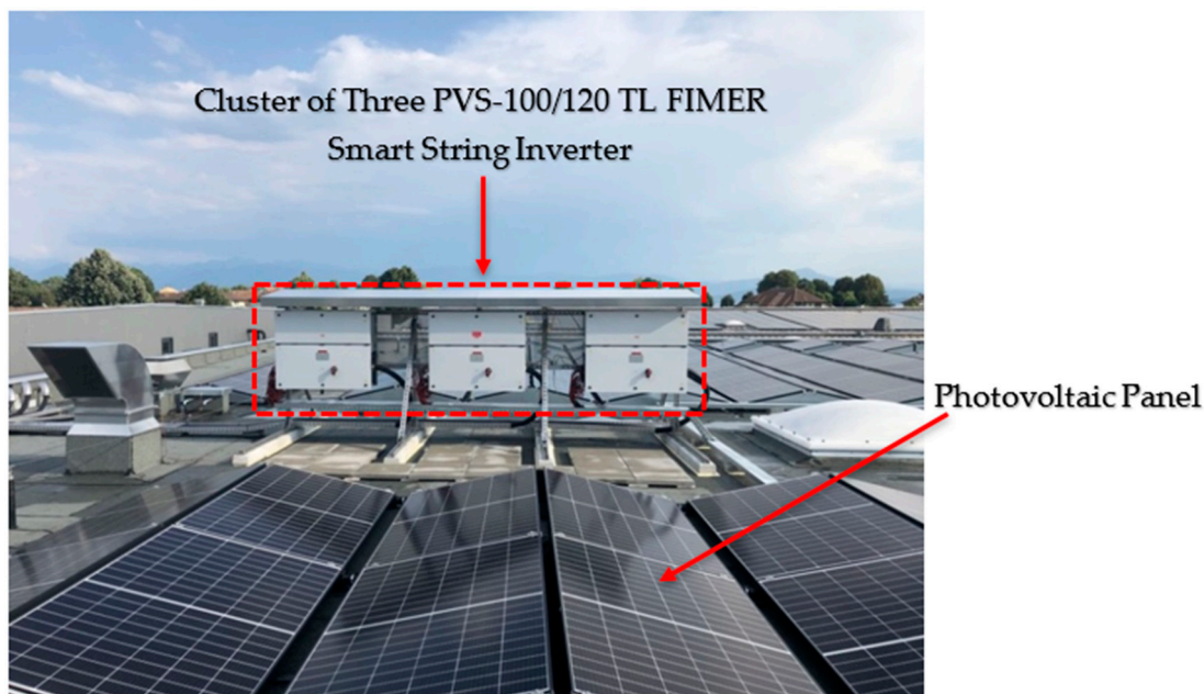
Figure 1. Photovoltaic (PV) installation of 280 KiloWatts (KW) featuring a cluster of three PVS-100/120-TL FIMER smart string inverters between Geneva and Lausanne, Switzerland. Photo courtesy of KDISOLAR.
