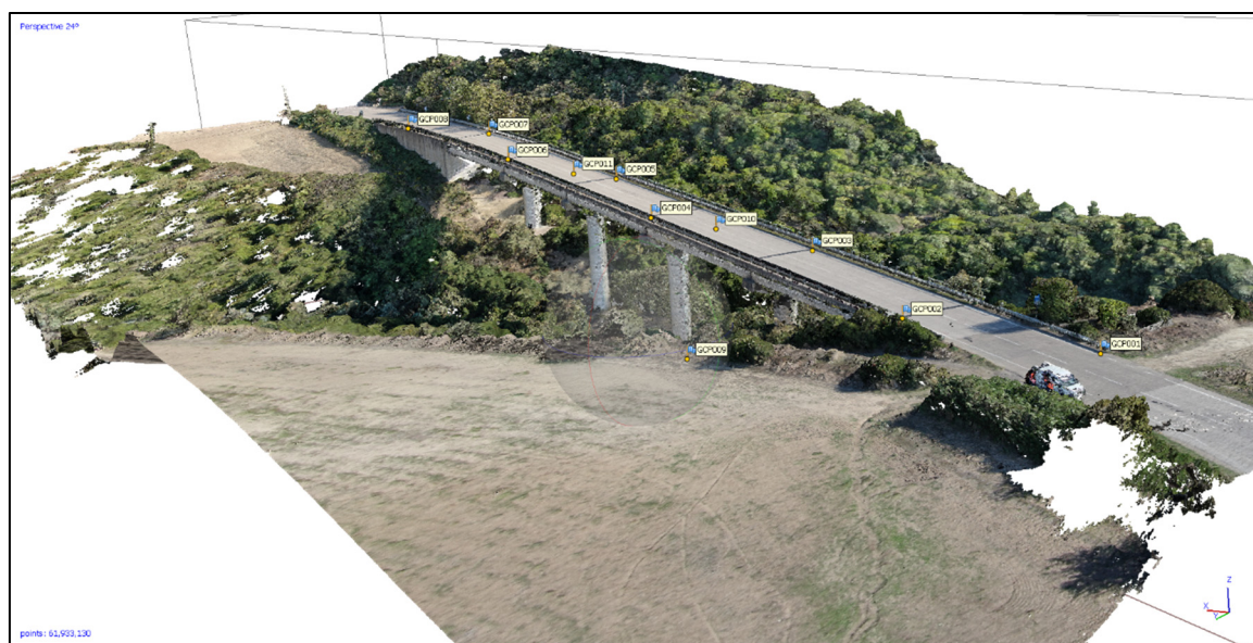
Figure 7. View of the obtained dense point cloud and GCPs/ICPs placement along the structure.
