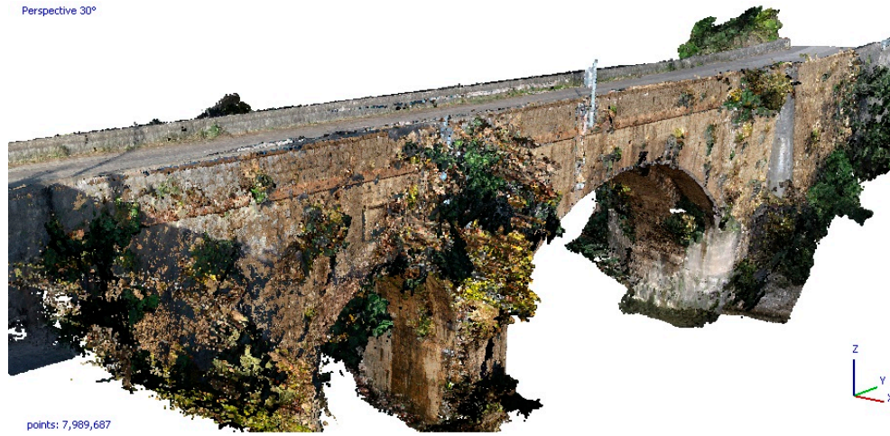
Figure 8. Three-dimensional point cloud of San Cono bridge (visualization in Agisoft Metashape software).
