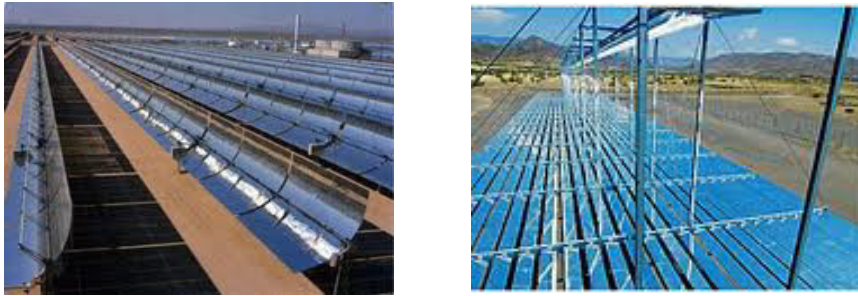
Fig. 1. Line focusing systems: Parabolic Trough (left) and Linear Fresnel (right).
