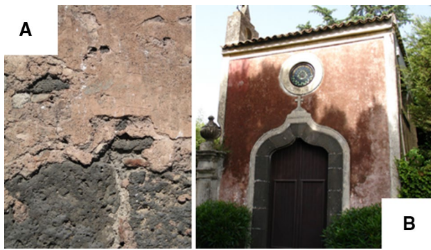
Fig. 3 a Detachment of mortar based on ghiara; b Original plaster application in San Salvatore church in Viagrande, Catania, Italy
