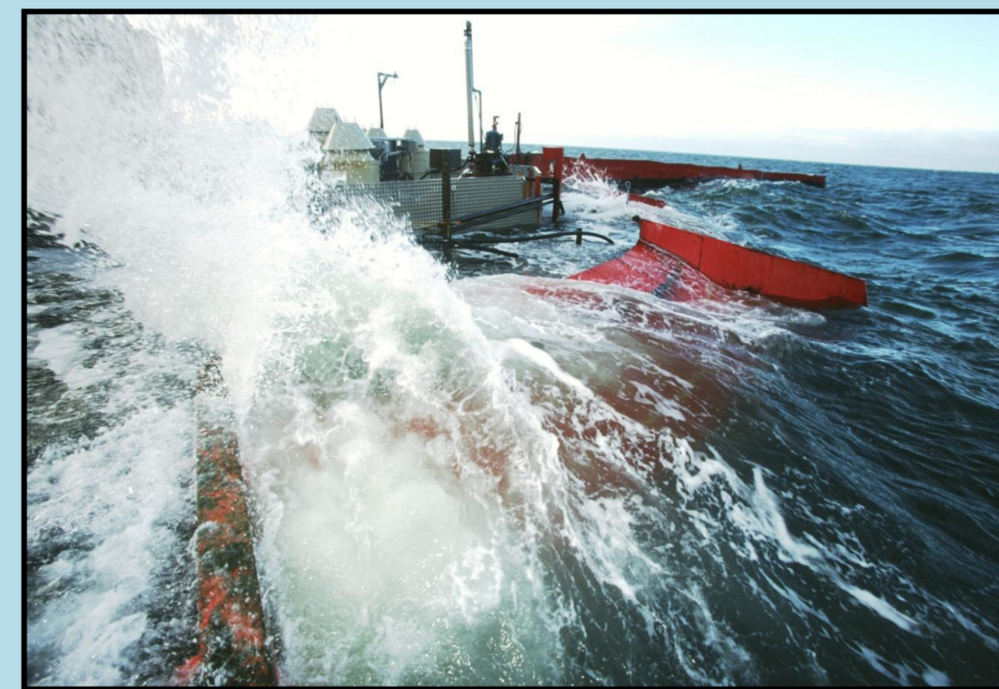
Fig. 4 – The Wave Dragon 1:4.5 scale prototype in action
