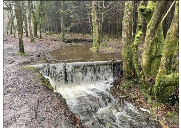
Fig. 1. Example of channel-spanning ELJ in a headwater stream (Nant Drysiog, Wales, UK, 16th February 2022).
