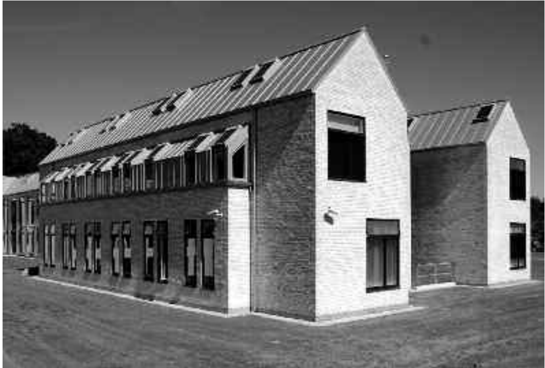
Figure 6 VKR Holdings headquarters, Hoersholm, Denmark, Hvidt & Mølgaard Architects (2007). Spatial proportioning creates high levels of well-distributed daylight. This provides a good working environment, low prima- ry energy consumption, and no need for mechanical cooling.
