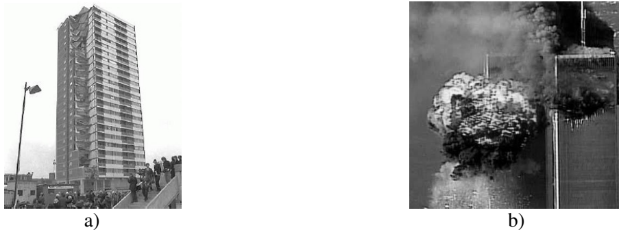
Figure 5.1: Structural collapses of buildings: a) Ronan Point building partial collapse; b) Twin Towers total collapse after terrorist attack
