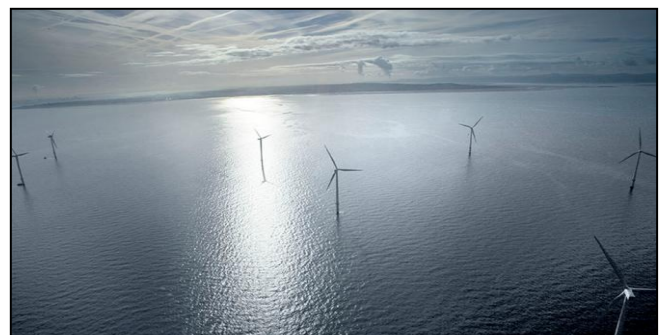
Figure 1 Large offshore wind farm with widespread MV submarine cable network.
