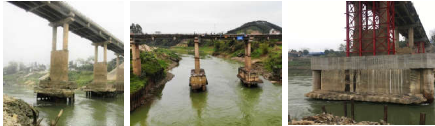
Fig. 4. Bridge foundations: from 1984-2013 (left); b. from 2014-2019 (middle); and c. 2020-current (right).
