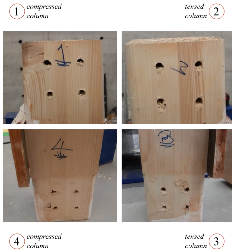
Figure 17: TREP3 test – Highlight of the damage in the joint holes of the timber columns.
