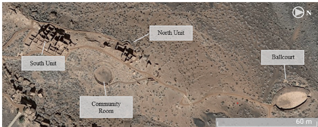
Fig. 8. Satellite view from Google Earth of the Wupatki Pueblo (South and North Units, Community Room and ballcourt).
