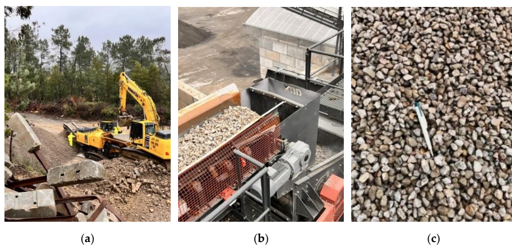
Figure 4. RCA processing: (a) crushing; (b) screening; (c) stocking.
