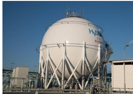
Figure 15 – Example of a spherical liquid hydrogen storage tank (Kyodo, 2023).
