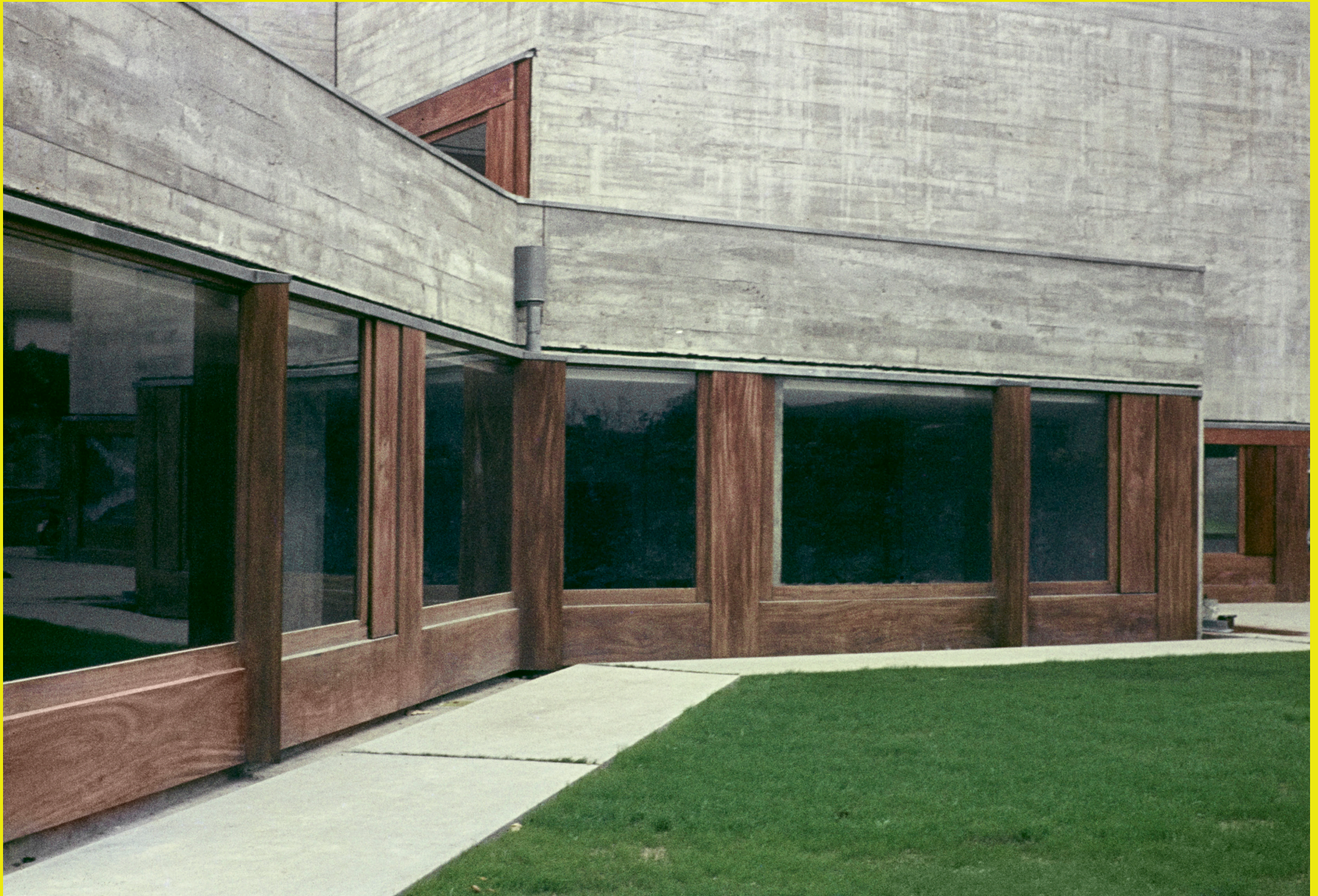
3. Lordelo do Ouro Cooperative Building, Porto; rare colour photo that illustrates its original features and condition as built by Álvaro Siza's (Jorge Gigante 1967, collection and courtesy of the author's family).
