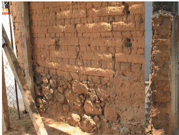
Figure 6. Typical adobe configuration in a house in the municipality of Tlayacapan.
