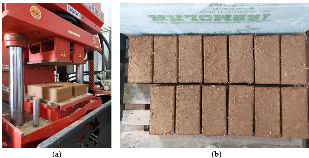
Figure 5. (a) Freshly manufactured blocks and (b) batch of blocks (mixture WS15) ready for curing.
