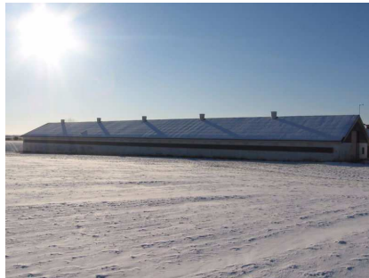
Figure 10.1: A Full Scale Poultry Stable Located in Syvsten, Denmark
