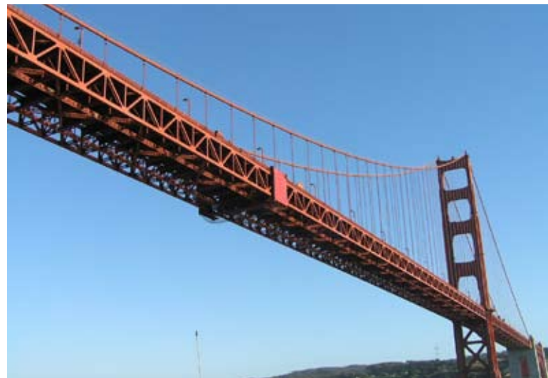
Golden Gate Bridge, San Francisco
