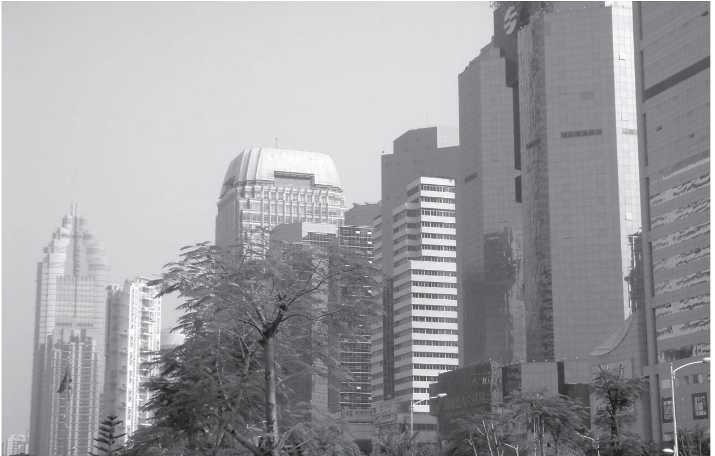
Fig.7: The continuous construction of sky scrapers (Photo: Gitte Marling)
