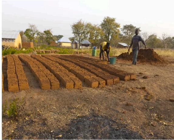
Fig. 2. Reddish Clayish soil used for plaster and blocks preparation in Wa, 2022 (photograph by the authors).
