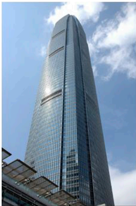
FIGURE 5 Technological advances in structural solutions and new materials (Two International Finance Centre).
