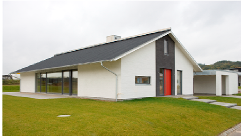
Figure 1. The studied passive house. Façades towards south and east.
