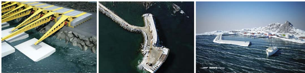
Figure 12. Different WECs on Breakwaters, from the lf:ConvOn, OWC, SSG.
