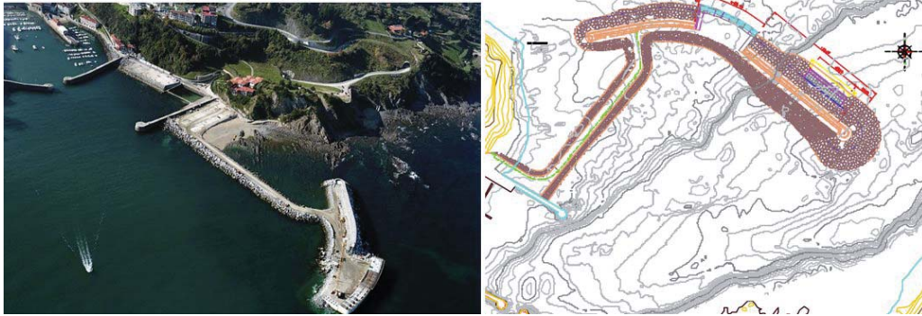
Figure 11. Mutriku OWC breakwater.
