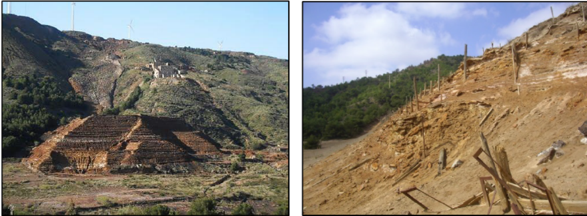
Figure 2.12. Left: abandoned tailings pond “Belleza”. Right: remaining wood poles used to increase the height at “El Lirio” tailings pond.
