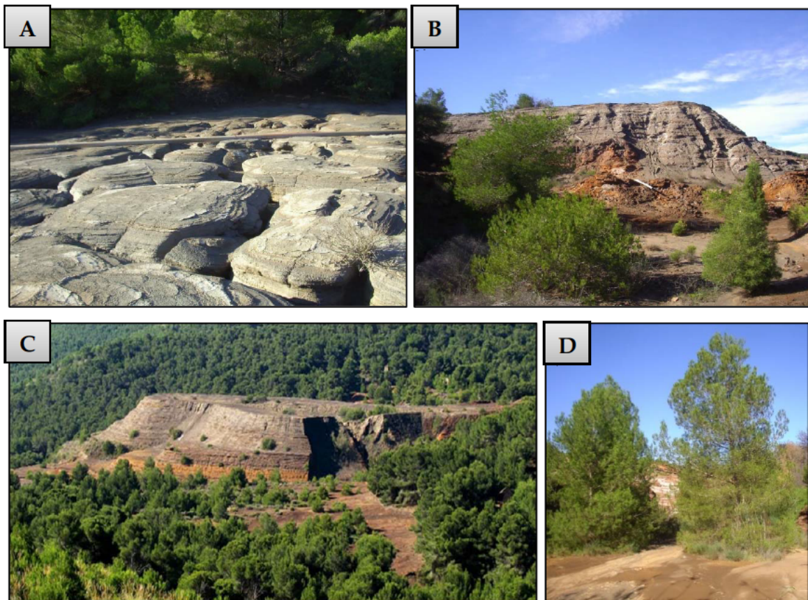
Figure 2.17. A) Surface erosion and cracks on “Agustin” tailings pile. B) Slopes erosion at “Agustin” tailings pile. C) Landscape impact of “Mercader” tailings pile. D) Mine wastes from tailings covering a close riverbed.
