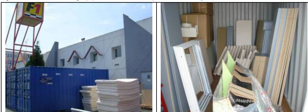
Figures 25: Containers storing equipments and materials. (Foto: Frédéric Bougrain).
