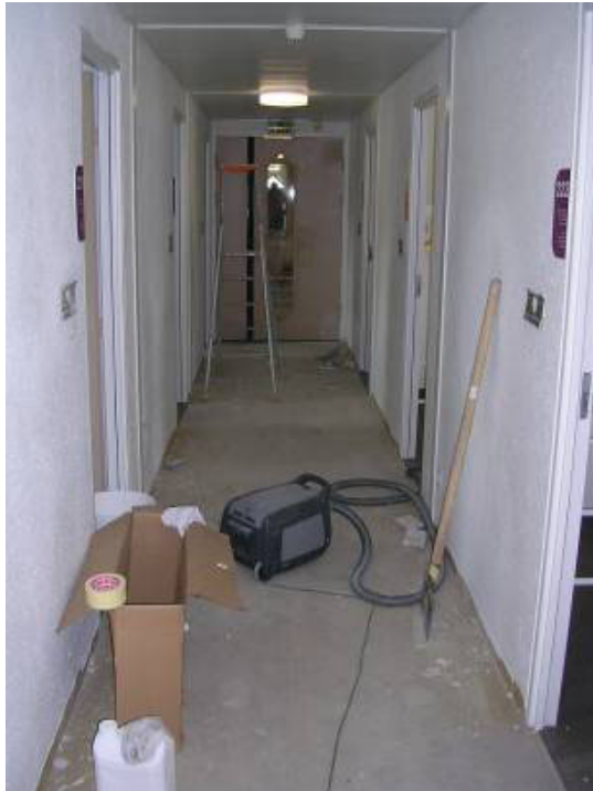
Figures 27: Renovation works. (Foto: Frédéric Bougrain).
