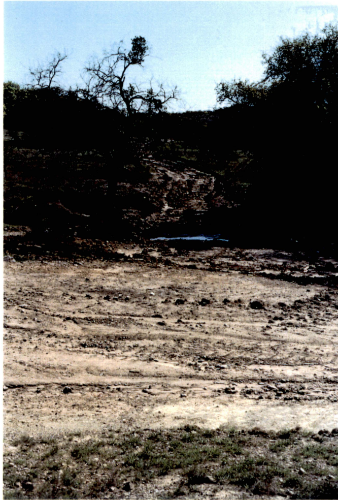
Figure 15. Photograph of road across flowing stream. Runoff from heavy rain will wash abnormal amounts of sediment into stream from defoliated areas.
