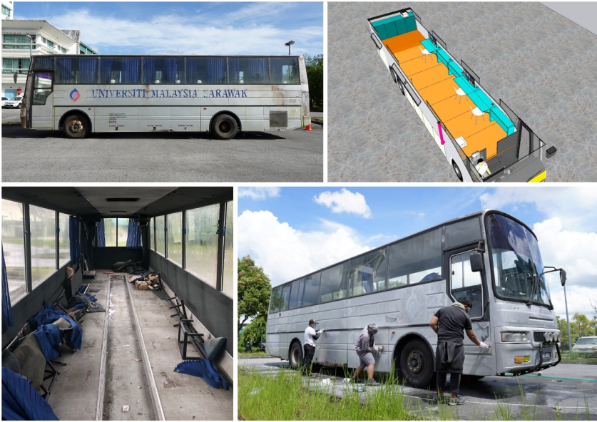
FIGURE 2 Clockwise from left: Delivery of donated bus, design concepts for the proposed interior design an initial exterior preparations. Work begins on the replacement of the flooring ahead of the internal refit.
