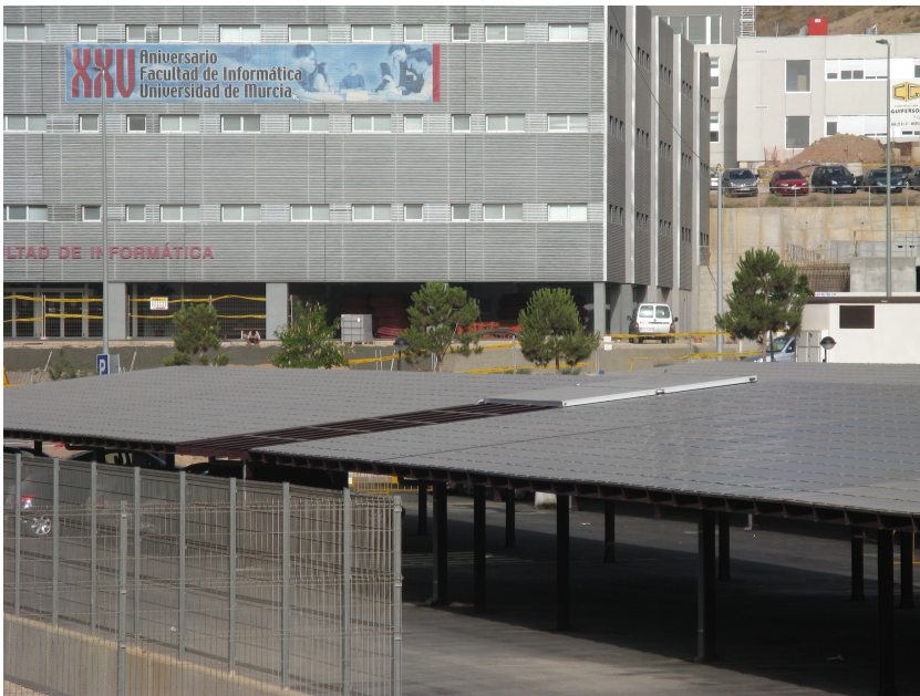
FIGURE 2.1 222KW p CDTE PARKING INTEGRATED GRID-CONNECTED FACILITY
