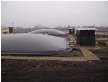
Fig 1: CHP biogas plant 160 kW e +300 kW th at farm Agro-Oven (15 thous. pigs), Ukraine. Design of BTG, the Netherlands.
