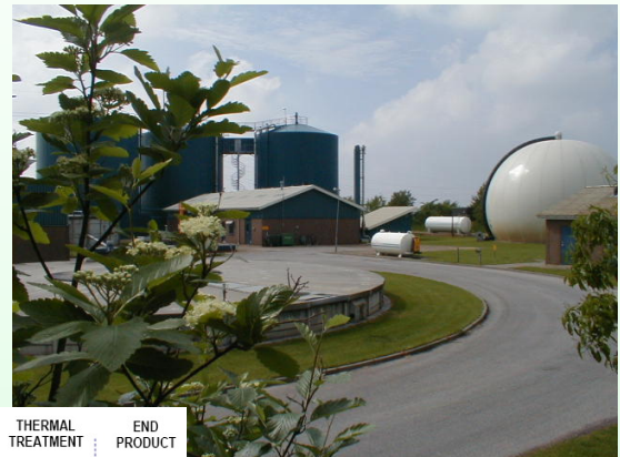
Ribe Biogas Plant
