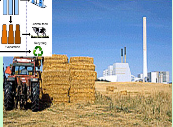
Studstrup Power Plant
