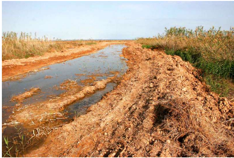
Photo 2.2. Channeling of the Rambla de Miranda in September 2003.
