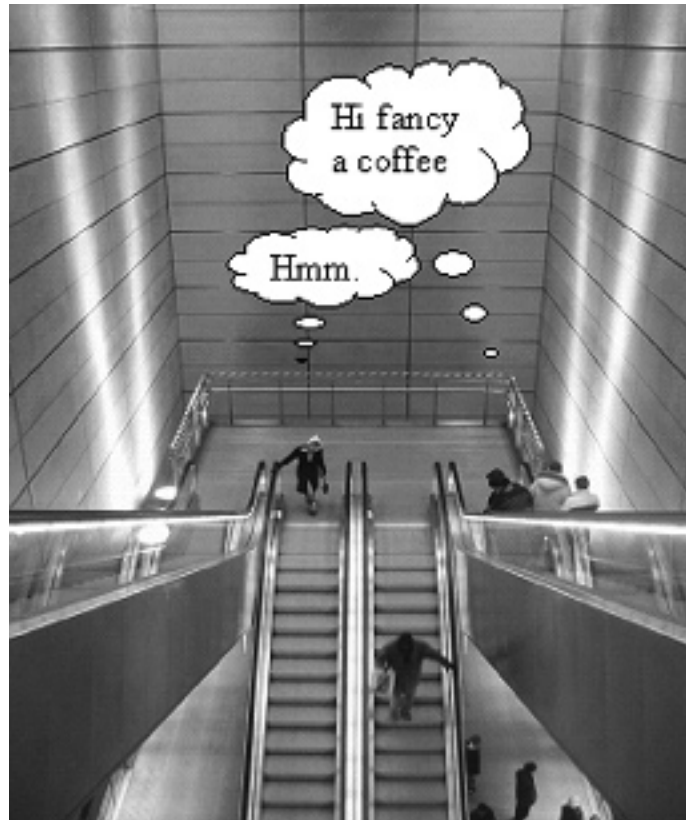
Figure 11. Escalator at the Copenhagen Metro
