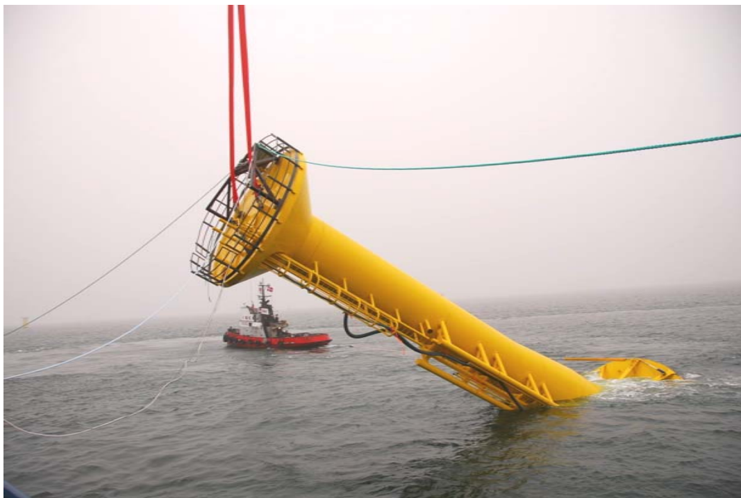
Fig. 6. Offshore installation of a monopod bucket foundation, Denmark, 2009.
