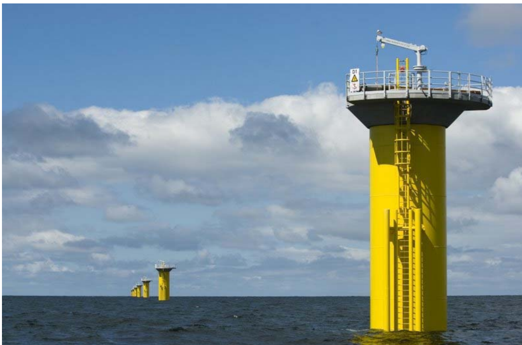
Monopiles at Horns Rev 2 Offshore Wind Farm, Denmark
