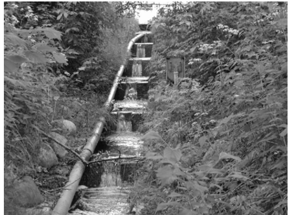
Figure 2 - Photograph of the fish ladder (July 2001) [2]
