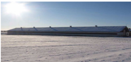
Figure 1 A Full Scale Poultry Stable in Denmark
