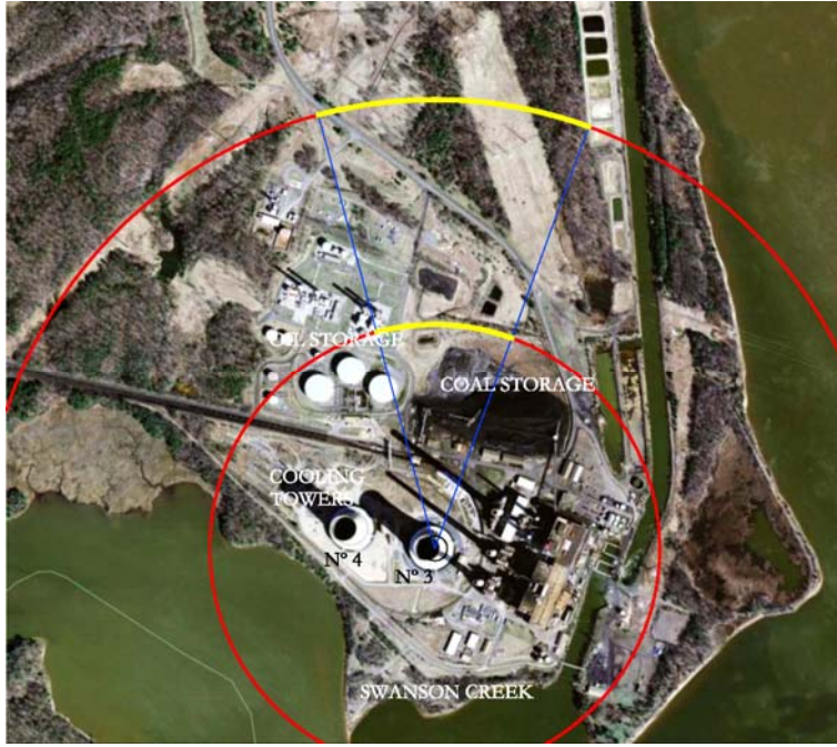
Figure 4: Sampling arrays at Chalk Point cooling tower number 3.
