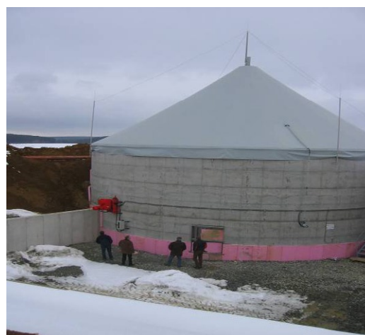
Figure 2. Fermenter No. 2 at Strem biogas plant. Insulation was not completed because this mesophilic fermentation process generated a surplus of heat surpassing that needed for keeping the process temperature constant. Inoculum at this biogas plant was cow manure but, after start-up, the feedstock was almost exclusively maize silage. Photo JBHN, 03/05-2005.
