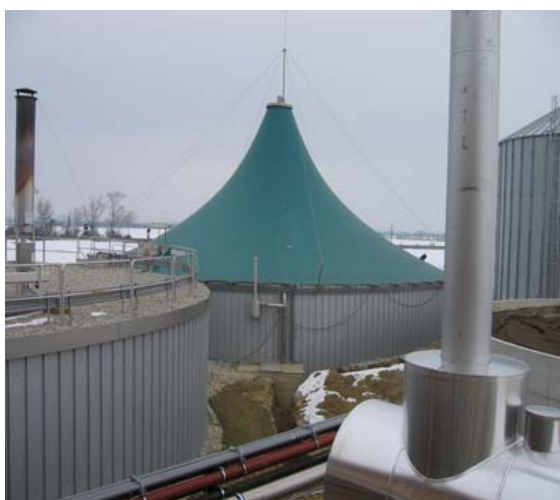
Figure 1. Reidling biogas plant. Fermenter No. 1, flat-roofed fermenter in extreme left field of view, has been in full operation as the main fermenter for one year. In the centre part of the photo is Reidling fermenter No. 2, which was set in operation in February 2005. Photo JBHN, 03/05-2005
