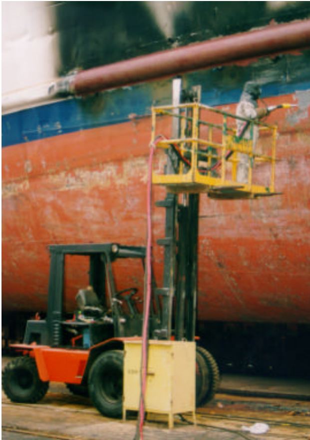
Figure 1. Grit blasting for hull cleaning.
