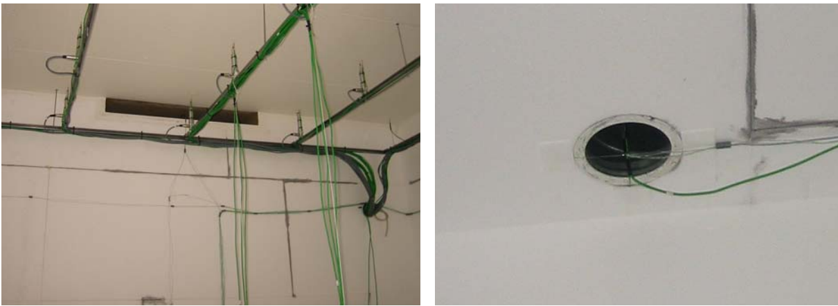
Figure 6. Ventilation openings. Left: Opening used as air inlet for mixing ventilation and outlet for displacement ventilation. Right: Outlet opening for mixing ventilation.
