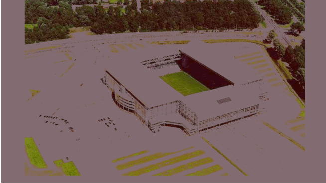
An innovative solution for stadiums: A sliding pitch to move the grass outside the stadium. Source: Frits Scheublin, BAM, The Netherlands
