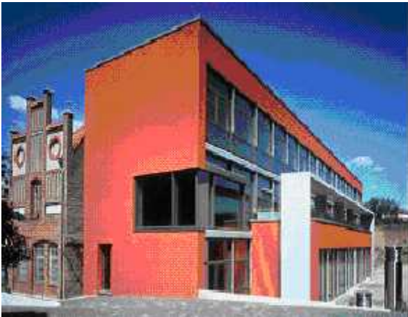
Figure 3.6 – The Centre for Sustainable Building (ZUB) in Kassel, Germany (De Carli et al. 2003)
