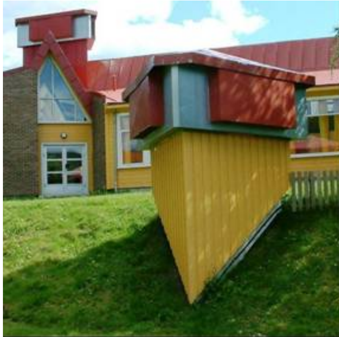
Figure 4.8. ETAHE's intake tower of Mediå school
