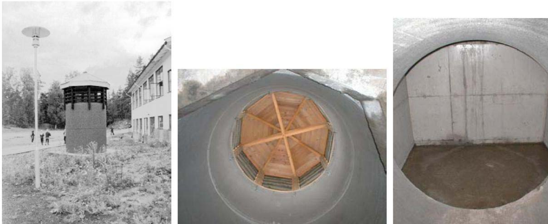
Figure 4.12. Jaer School air intake tower (Left: outside, Middle: inside looking up, Right: inside horizontally into base of the tower from the horizontal ETAHE duct.) (Schild 2002a).
