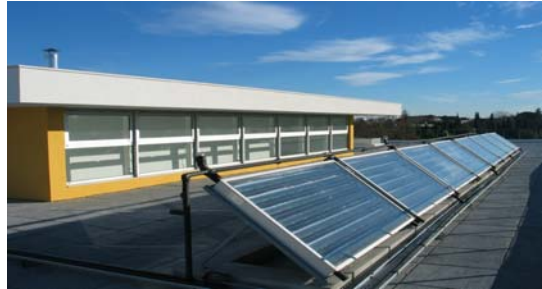
Roof window for ventilation and daylight and set of CPC solar collectors
