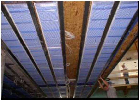
Heating and cooling panels, which are flown with cold water (cooling period) or warm water (heating period), product “RCS“
