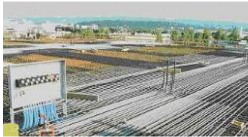
Installation of the TABS on site
