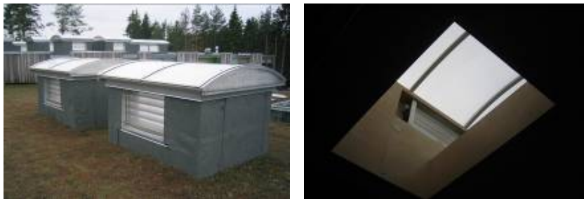
Skylights used for lighting and for air exhaust.
