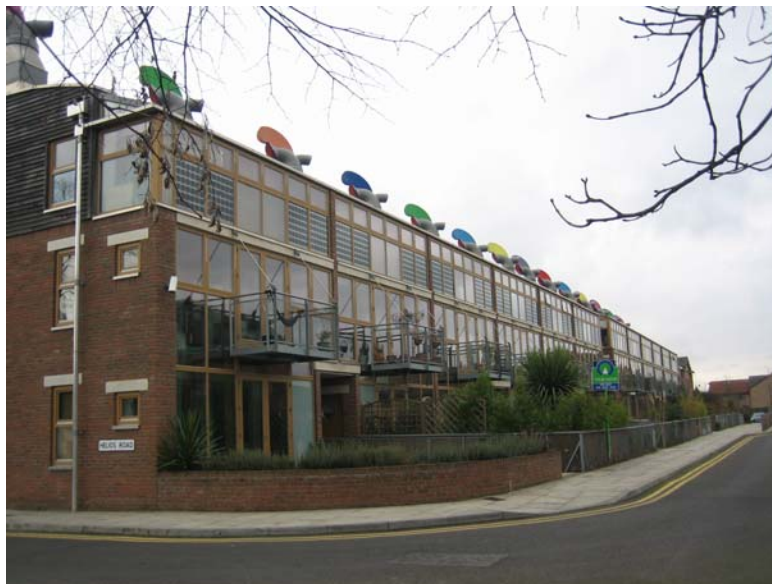
East facing façade with winter gardens and PV panels in the façade and on the glazed roofs of the winter gardens.
